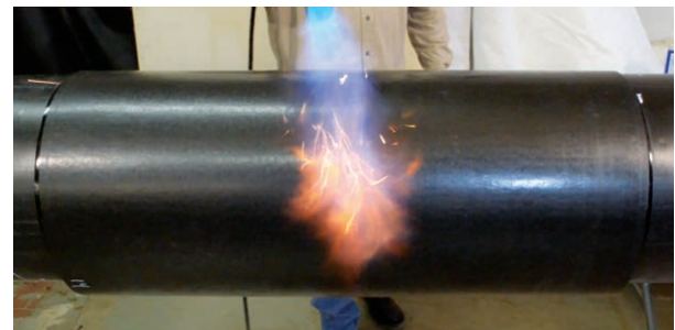
Heat shrinkable, HDPE full round rigid sleeve. Note: Sleeve must be slid on pipeline before welding the carrier pipe together.
