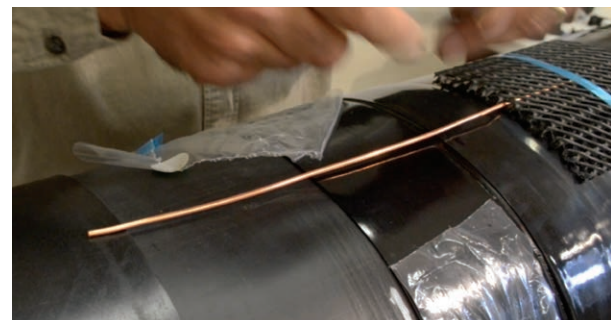
Waffle board and pipe for air testing of the joint.
