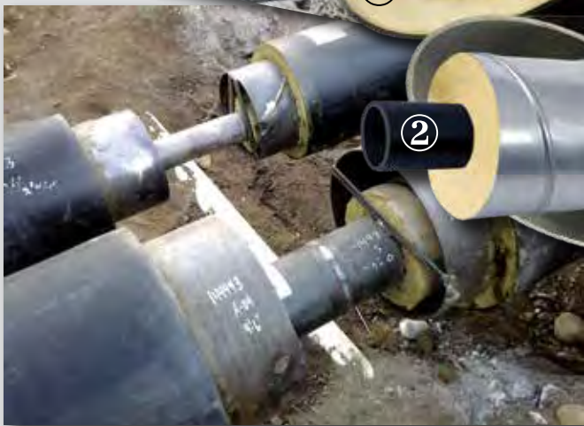
Rhinocoat® Hi Temp Conduit with 400°F Hi Temp Polyisocyanurate Foam Carrier Pipe Insulation
