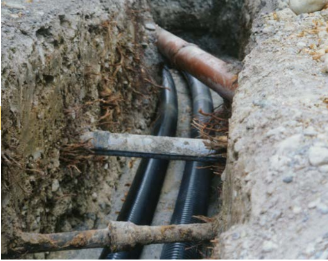
Rhinoflex flexible pre-insulated pipe easily follows the route and contour of the trench.
