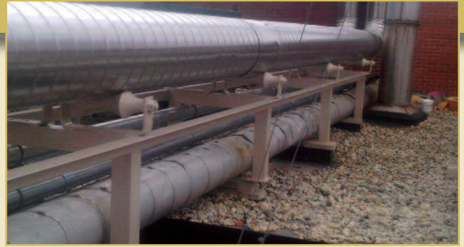
The picture above shows the Rovanco product on top and a field insulated pipe below. The labor and energy savings with Rovanco piping is substantial.
