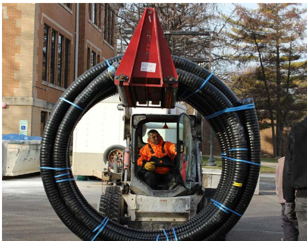
For larger coils, larger diameter pipe or lack of extra personnel, a RhinoRoller can be used to ease uncoiling process.
