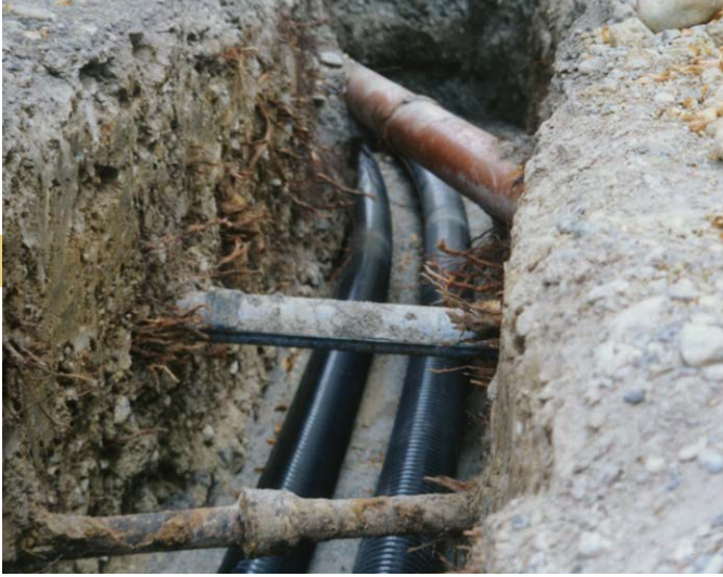
Rhinoflex flexible pre-insulated pipe easily follows the route and contour of the trench.
