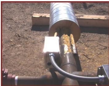
Piping can be ordered with a tube adding electronic heat trace capabilities to the system.
