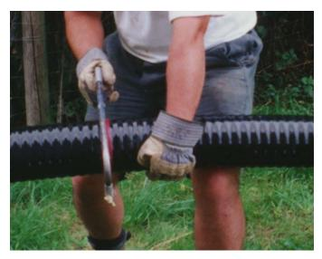
Rhinoflex can easily be cut to length with just a hacksaw. No special tools or equipment are required to install. Rovanco provides complete installation kits, accessory materials, installation instructions. No special training or skills are required.
