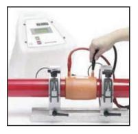
13. Connect electrofusion welding unit, using the red nipple to the red contact. Welding and cooling parameters are automatically detected. If not then scan bar code. If parameters still do not show then physically type in code.
