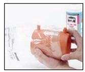
9. Remove PEX fitting and clean interior with denatured alcohol.
