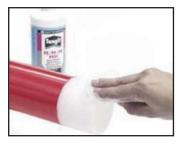
8. The scraping area must be free of dirt and oil. Clean the area with an adequate amount of denatured alcohol and allow the cleaning agent to completely evaporate.
