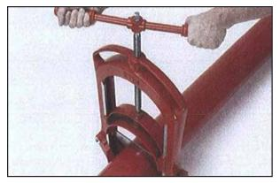
1. Cut the pipe into lengths of the required size with a square cut using a guillotine...
