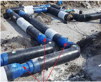
Wrap joints similar to this example
