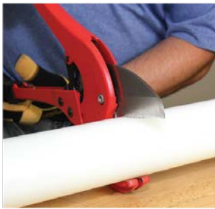
Figure 14: Cut pipe
