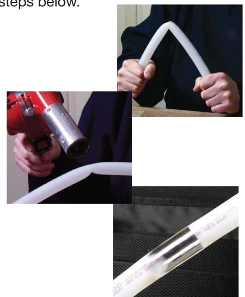
Figure 43: Reforming Kinked Piping
