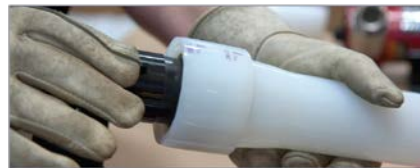
Figure 26: Insert fitting
