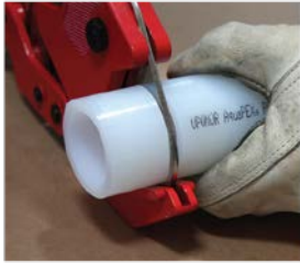
Figure 20: Cut pipe
