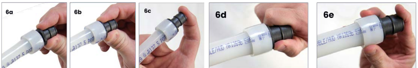
Figures 6a-6c: Inserting ProPEX fitting into 1/2" Uponor PEX fitting
