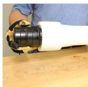
Figure 19: Insert fitting
