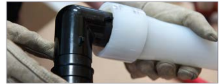
Figure 27: Ensure piping and ring seat against shoulder of fitting
