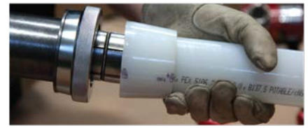
Figure 24: Rotate head
