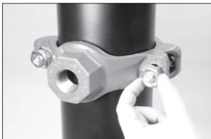
**4. INSTALL REMAINING BOLT/NUT:** Insert the remaining bolt. Thread a nut onto the bolt finger-tight. Ensure that the bolt track heads seat properly in the bolt holes.
