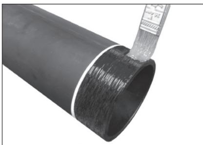
**4. LUBRICATE PIPE END:** Apply a thin coat of lubricant to the pipe end, from the end of the pipe to the paint mark made in step 3.
