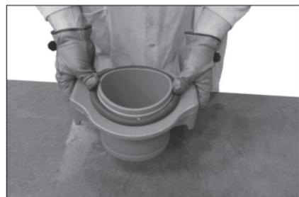
**5. INSTALL O-RING:** Press the o-ring into the groove on the underside of the spigot housing. Do NOT place the o-ring on the pipe and then attempt to push the locating collar through it. This may push the o-ring into the hole, and will prevent proper sealing.
