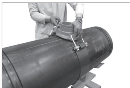
**8. ATTACH STRAP:** On the opposite side of the pipe, pull the second U-bolt up and hook it over the second retaining gusset of the spigot housing.
