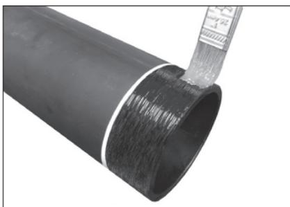
**4. LUBRICATE PIPE ENDS:** Apply a thin coat of lubricant to the HDPE pipe end, from the end of the pipe to the paint mark made in step 3.
