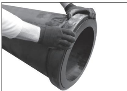
**3a. POSITION GASKET:** Position the gasket over one pipe end. Verify that the gasket does not overhang the pipe end.
