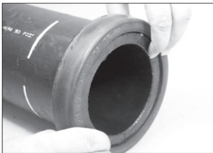
**5. INSTALL GASKET:** Install the gasket over the pipe end. Ensure that the gasket does not overhang the pipe end.
