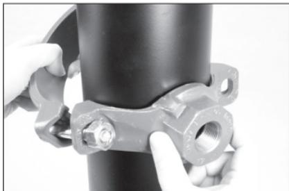
**3a. INSTALL HOUSINGS:** Rotate the lower housing so that it is positioned approximately 90° to the upper (outlet) housing, as shown above. Place the upper (outlet) housing onto the face of the pipe in line with the outlet hole cut into the pipe. Rotate the lower housing around the pipe.
