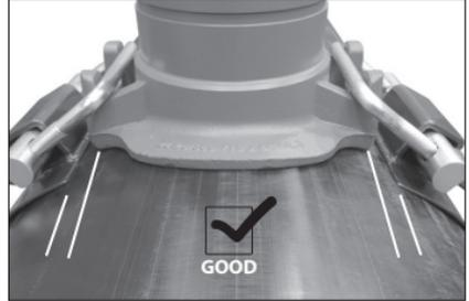
**11. INSPECT ASSEMBLY GAPS:** Ensure that the spigot housing is an equal distance from the strap on each side. If the strap hardware does not grip the housing evenly from both sides, the assembly may be pulled out of alignment, causing the housing to angle into the hole and creating improper compression of the o-ring.
